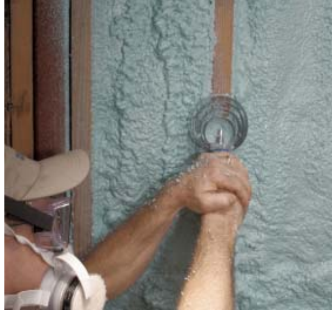
Figure 5. Open-cell foam, which expands to about 100 times its liquid volume, typically has to be trimmed flush to framing members — an easy task, since the foam is so soft. Because of its lower expansion rate and higher R-value per inch, closed-cell foam doesn't usually have to be trimmed. When it does, as in this shallow rafter bay (left), the author's crew uses a scraper — in this case a horse curry comb — to clean the framing in preparation for drywall (right).
