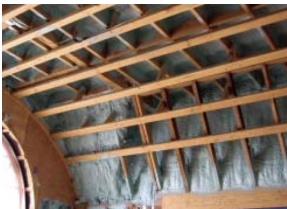
Figure 4. This barrel ceiling (above) would be difficult to insulate and seal with traditional materials. It's an ideal candidate for spray foam, which conforms to its irregular surfaces (left).
